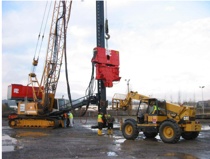
Figure 2. Supporting crane, pump, and vibration machinery.
