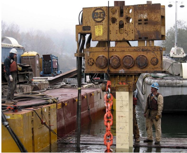
**Figure 1. Vibratory driver.** An APE Model 200 vibratory driver/extractor drove all piles during construction. It is shown driving the primary segment of pile S3U.
